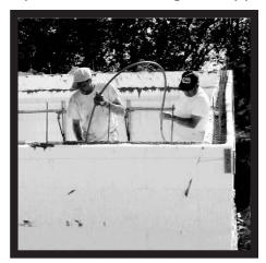
The rule of thumb for internal vibration is fast in and slow out, always moving, with a withdrawal rate of approximately 3" (76 mm) per second.
