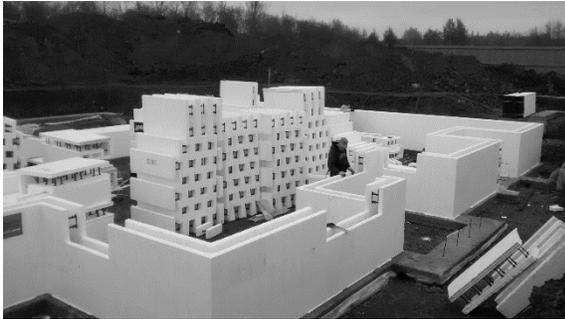
Make note of window heights and plan to cut in the window bucks accordingly. Mark them out on the wall forms and cut the sections out to fit the bucks, then proceed to block up to the bucks and continue building the wall.
