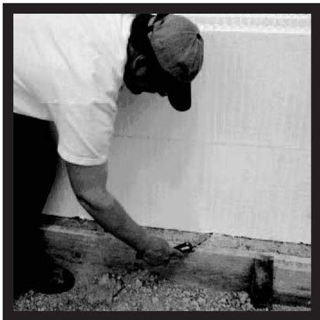
**STEP 7:** Confirm that the wall is straight and level. If adjustment is required, shim or trim the bottom of the wall until level is achieved. Humps or dips will compound each row and cause the wall measurements to be skewed later.
