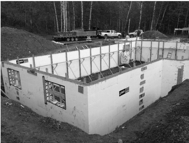
If you need to stack identical corners in subsequent courses, you will need to provide additional form support where the stacked joints are created.
