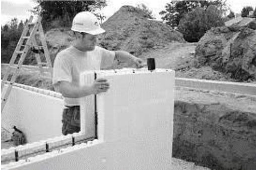
**STEP 2:** Fasten every corner end-to-end to adjoining forms using zip ties or horizontal hooks, and/or adhesive foam.
