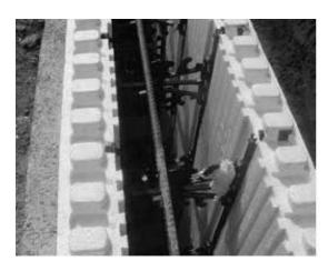
Reinforcement around windows and doors needs to be installed as required. Always check ICF manufacture engineer specs to ensure proper size, amount, and location of rebar is being placed.
