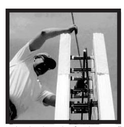
**STEP 1:** Install vertical rebar, as required, after all courses and horizontal reinforcement have been placed.
