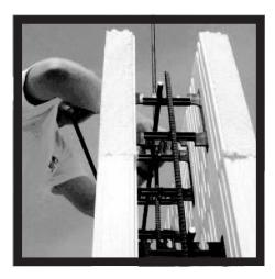
**STEP 1:** Horizontal rebar, sized as required, should be placed in the wall as each course is installed.
